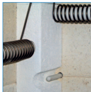
Thermocouple in protec- ted position
